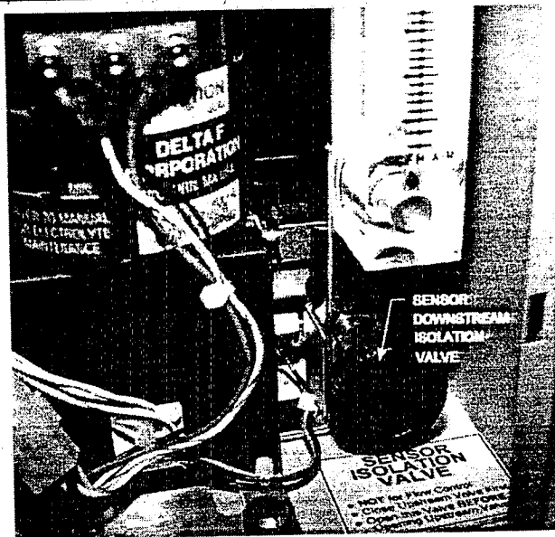
Figure 6-2. Sensor Downstream Isolation Valve
